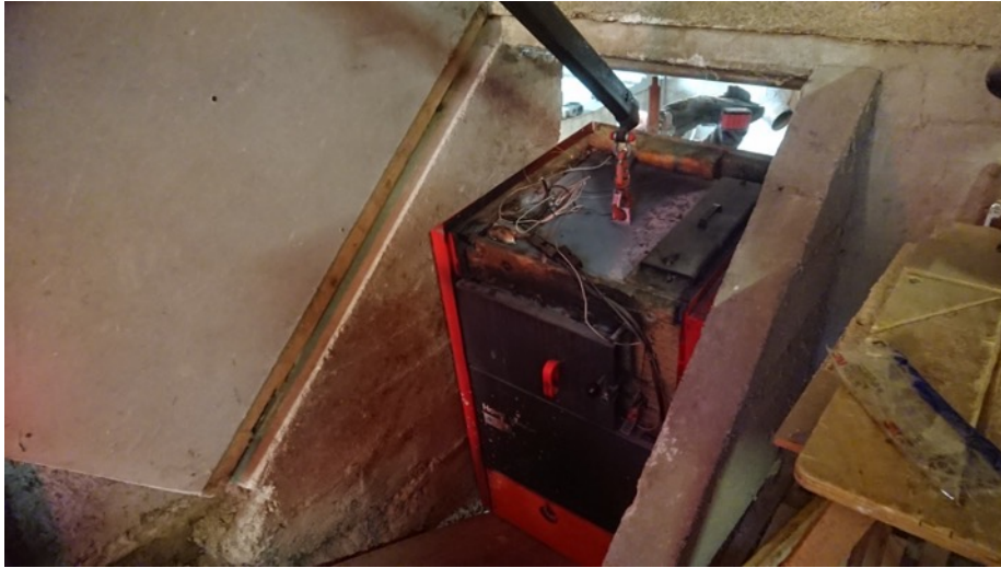
Demontage alter Kessel
